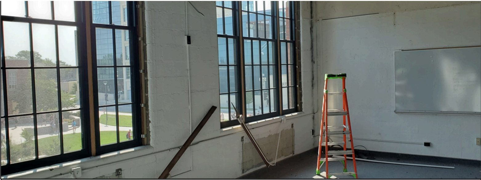
AF Classroom on east side of M&N (No more radiators)
